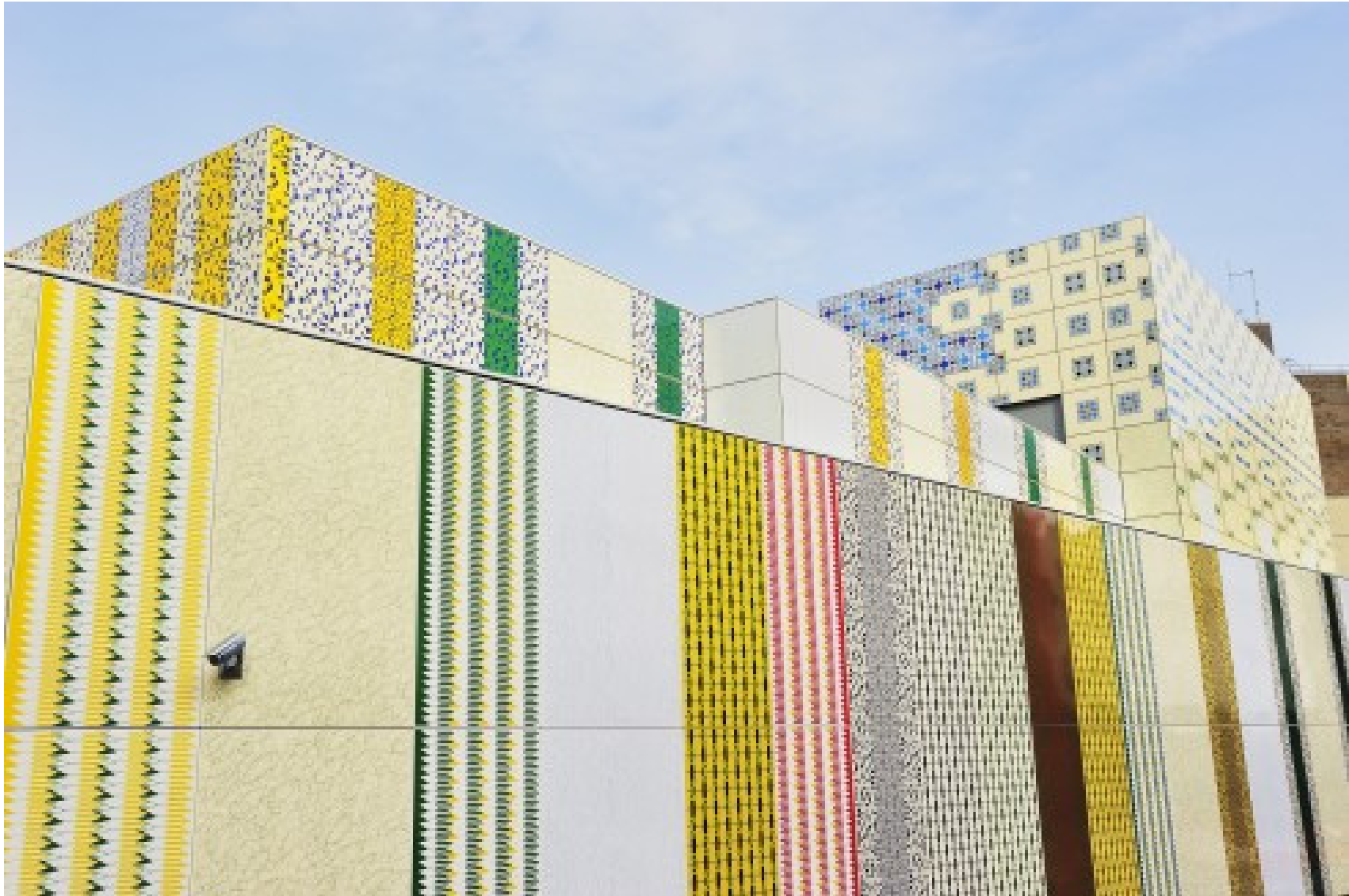
Wrapper, Jacqueline Poncelet, Edgware Road station, 2012 Photograph: Thierry Bal
